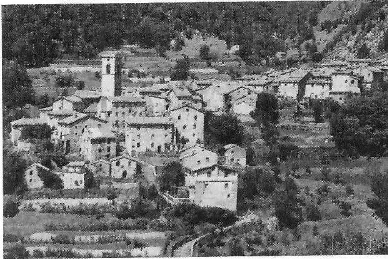
Vallico Sotto, viewed from the southeast.
